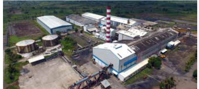
View of the 19.70 MW cogeneration plant
