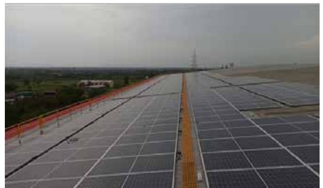
Rooftop Solar Panel: We have installed a 200 kW solar panel on our Godown top, from which we generate average 800 to 1,000 units/day, due to which we are saving Rs. 12,000/day in power costs.
